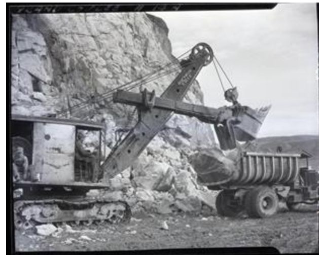
Original Caption: Washington, Coulee Dam - Power shovel and heavy duty truck really move rock. Local ID: 69-PWA-P-1994 (National Archives Identifier: 434070821 ).
