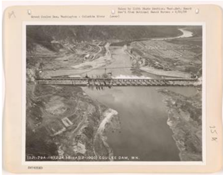
Photograph of the Grand Coulee Dam, taken by the 116th Photo Section, Washington National Guard. March 25, 1938. Local ID: 18-AA-134-25A (National Archives Identifier: 68151535 ).
