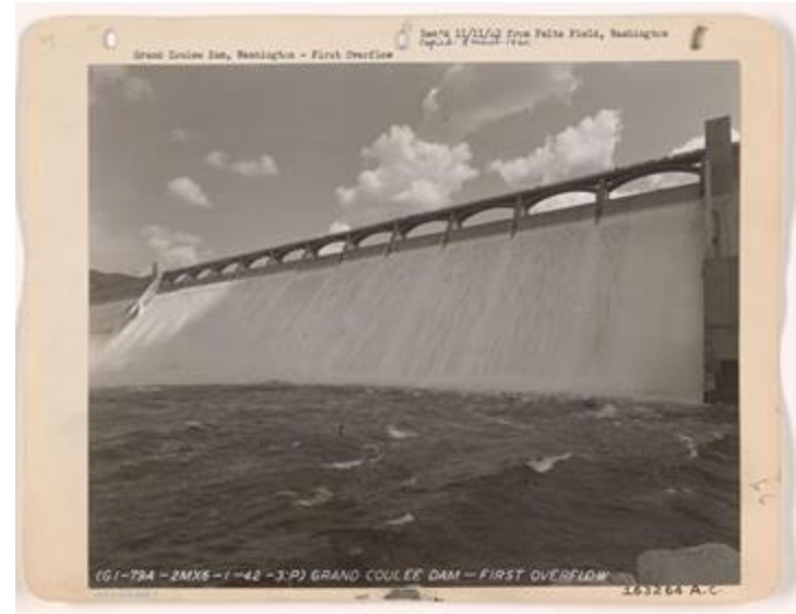
Photograph of the Grand Coulee Dam - first overflow. ca. June 1, 1942. Local ID: 18-AA-134-66 (National Archives Identifier: 68151569 ).
