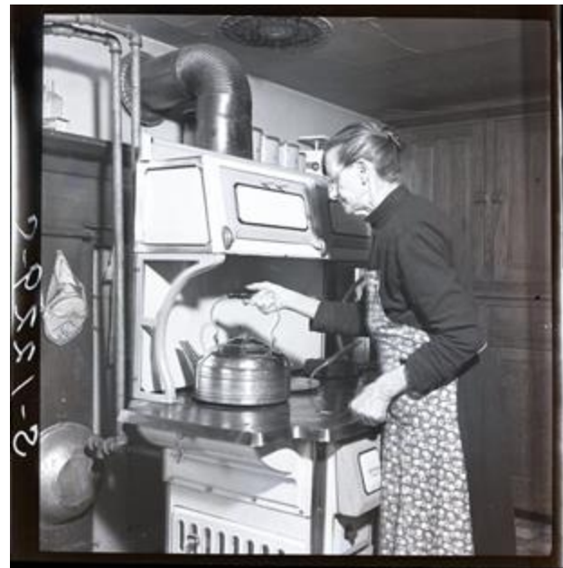
Photograph of woman at newly installed electric range. August 1938. Local ID: 221-G-1229 (National Archives Identifier: 432882302 ).
