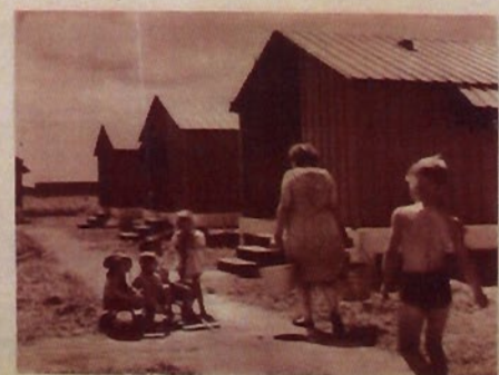
WATER IS EASILY AVAILABLE at the head of each shelter unit at the government camps.
