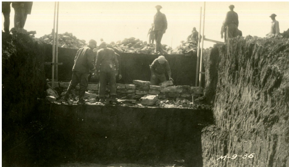
Above: Beginning double-drop dam on Strode(s) outlet. Narrative Report of S.C.S.-Mo-9 at Blue Springs, for 6th Enrollment Period, Oct. 1, 1935-March 31, 1936. Callaway County, Missouri State Office, Soil Conservation Service, Southeastern Region, Record Group 114, U.S. Department of Agriculture.
