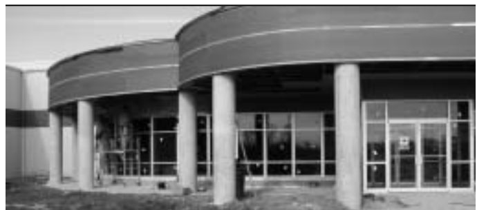
The new Dayton center under construction. (Photo by David Cornelisse)
