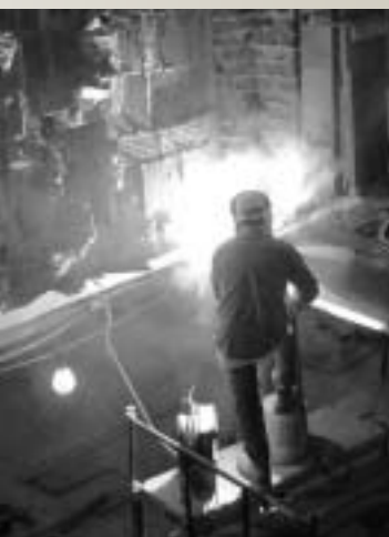
A welder works on an area where new elevators will be built in the National Archives Building in Washington, DC. (Photo by Earl McDonald)
