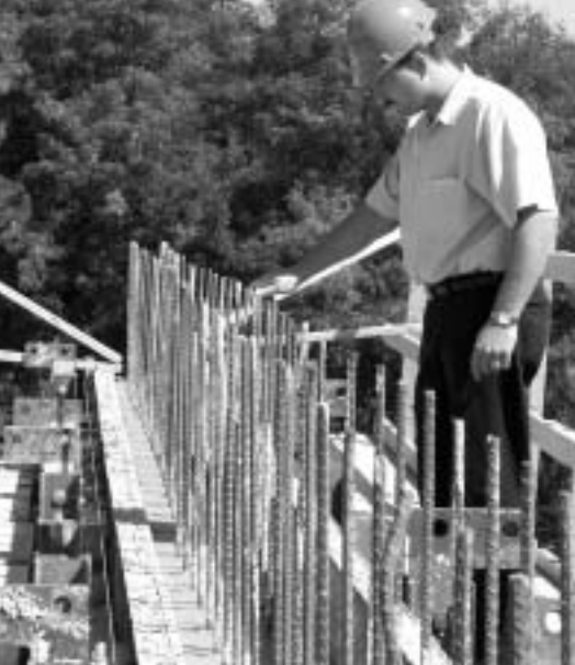
Facilities manager Mark Jonick views construction of a new wing to the Gerald R. Ford Museum in Grand Rapids, MI. (Photo by Donald Holloway)
